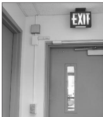
Typical applications for 500 & 700 Series Raceway.
