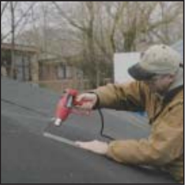
Weld Roofing Felt
