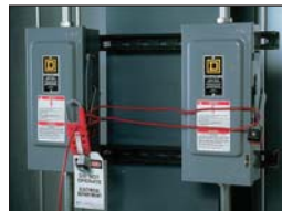
Lockout single or multiple electrical disconnects
