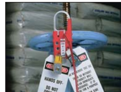
Lockout gate valves
